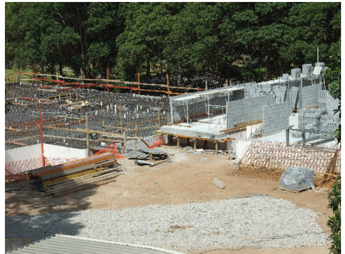
The new Weemala is on schedule for completion by mid 2011
